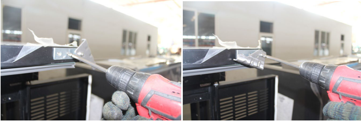
6.install the down hinge
